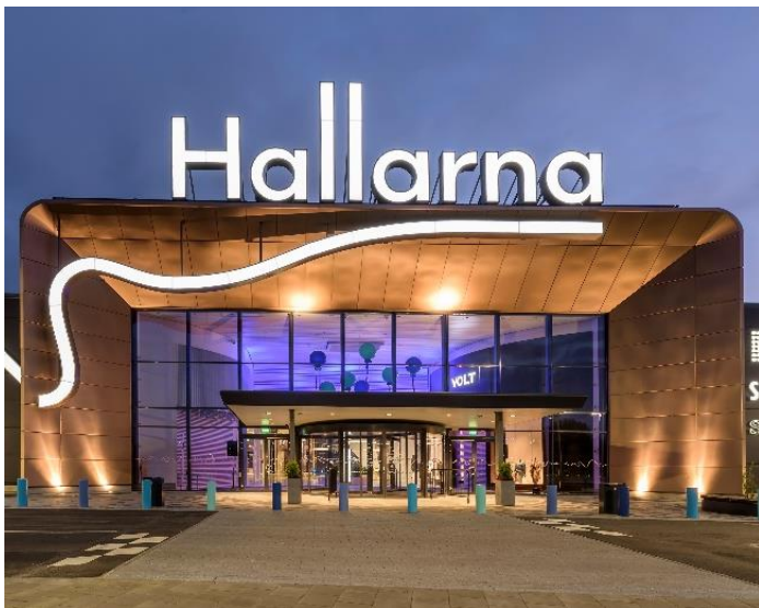
Entrance to the extended and refurbished Hallarna, Halmstad
