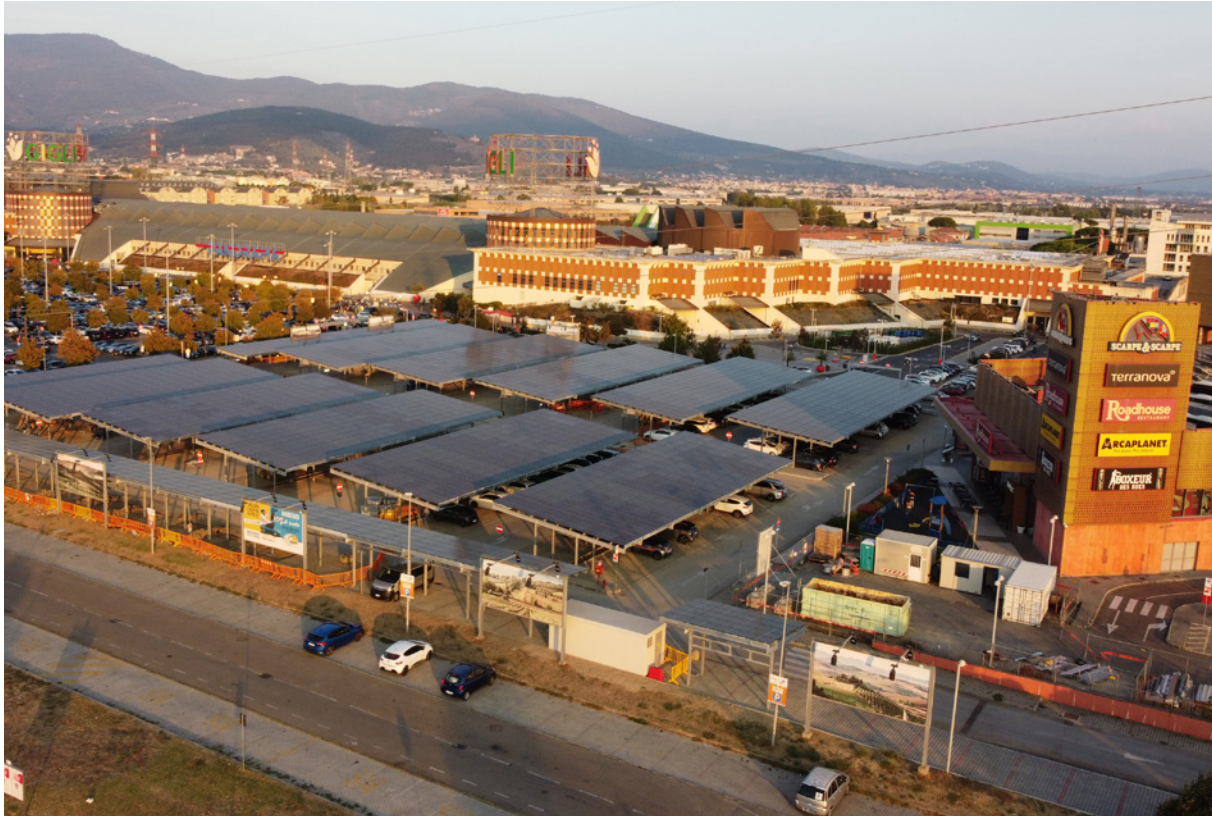
Solar panels at I Gigli on shelters covering 355 parking spaces
