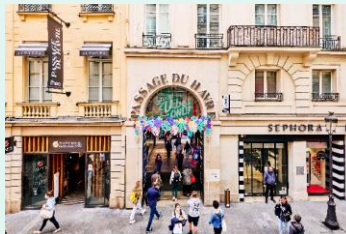
Passage du Havre, Paris, 50% office & residential completed in March 2022 for €57 M
