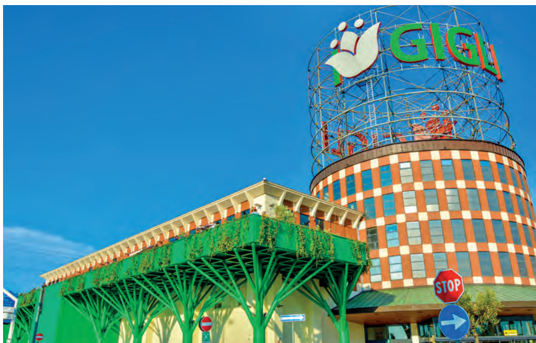
The new terrace at I Gigli.
