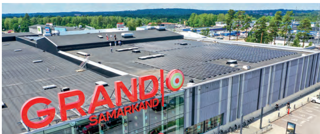
Solar panel roof installation at Grand Samarkand.
