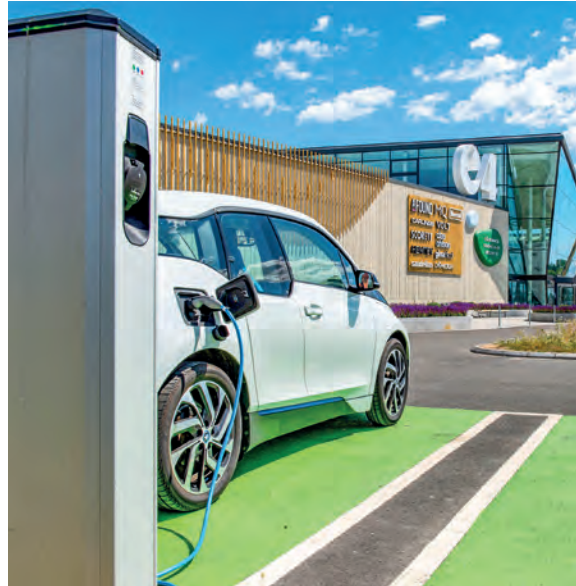
C4's electric car charging points.
